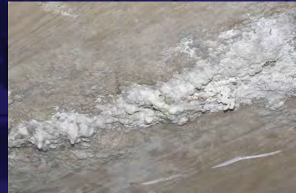
Picture 3: Efflorescence
