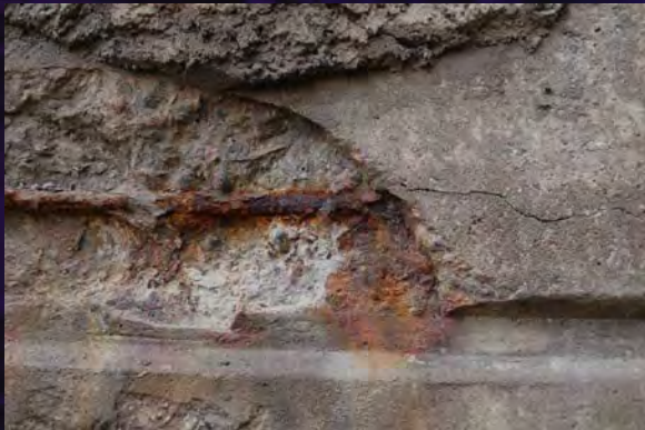
Picture 1: Corrosion
